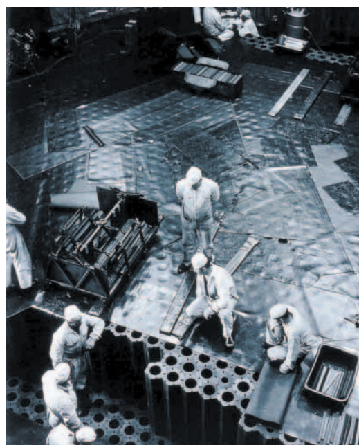
Graphite stack in a gas-graphite Uranium reactor
