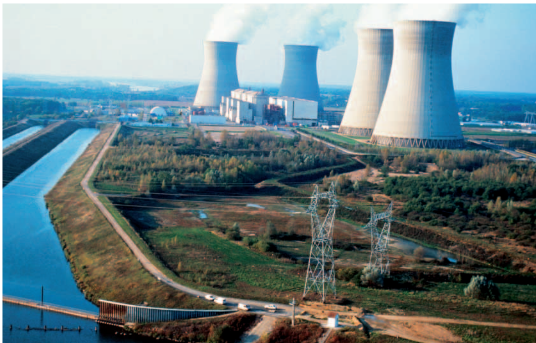
Dampierre-en-Burly nuclear power plant
