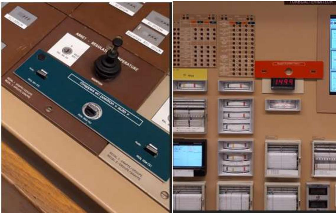
On the left, control rod switches in automatic position with plaque (green side) in place.
