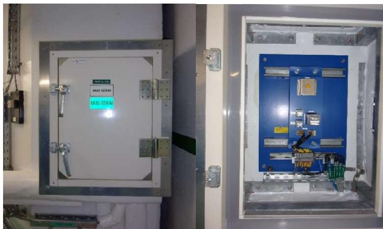
Installed Electrical Cabinet for opening of the pressurizer relief valves.
