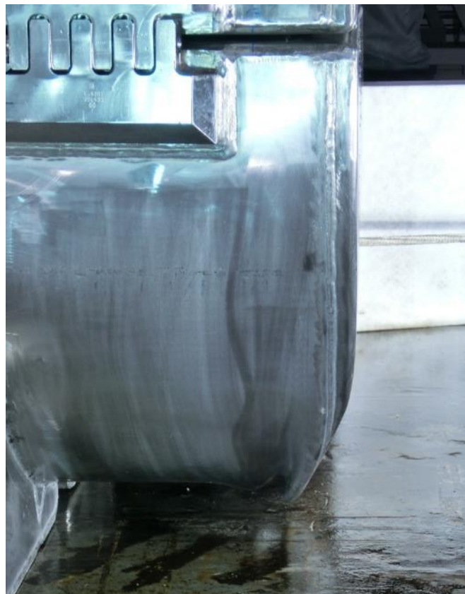
Figure 45: Sequence 2 - Deformation after the 1.2 m drop
