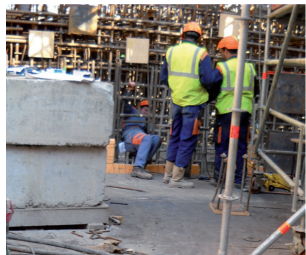
Positioning reinforcing bars on the EPR site – October 2009
