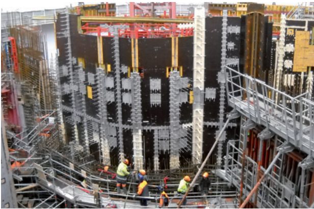
View of the concrete formwork of the EPR spent fuel pools – August 2010
