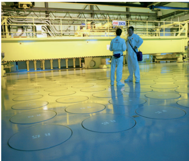
Interim storage hall of the vitrification facility R7, on the La Hague spent fuel reprocessing site
