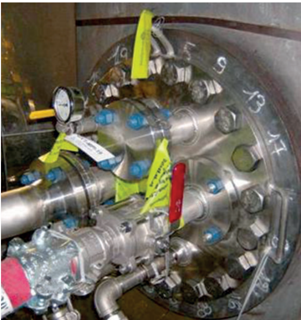
Installation of equipment during chemical cleaning of a steam generator
