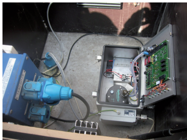
View of a seismic monitoring device (accelerometer) in an NPP
