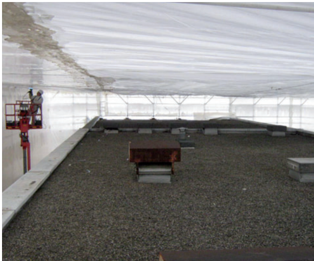
Installation of an internal lining for a decommissioning operation – STED Grenoble – February 2010
