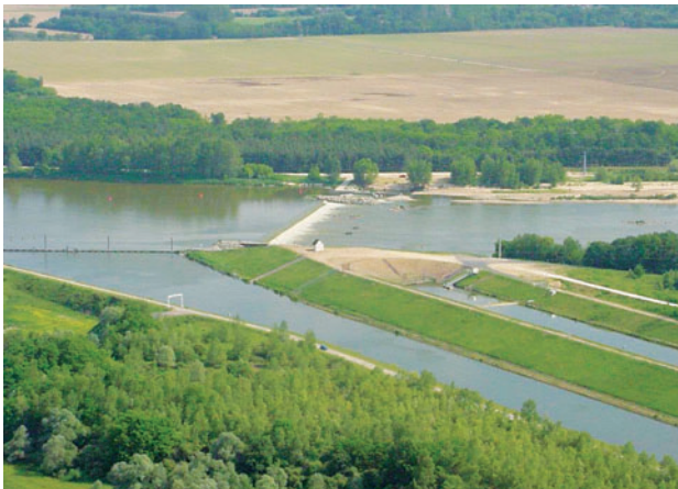
River Loire water take-off and discharge structures of the Dampierre-en-Burly NPP
