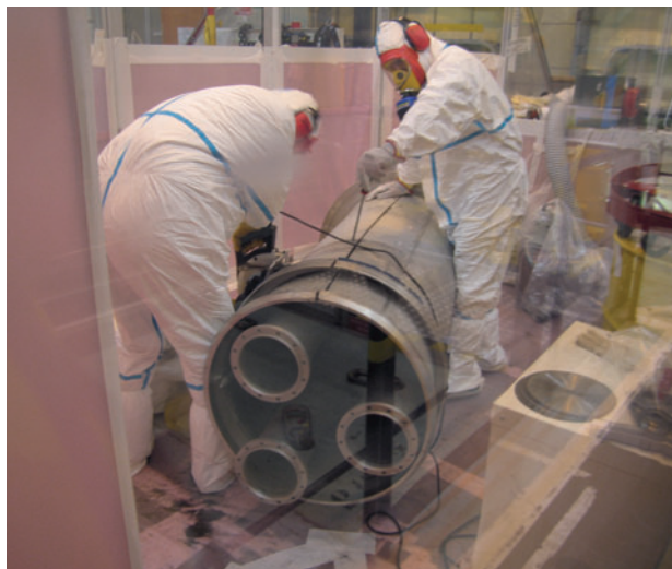
Cutting operation on an item of equipment of the PHEBUS experimental reactor at Cadarache
