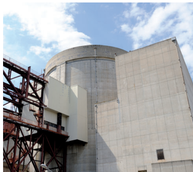
View of the concrete hull of a reactor building
