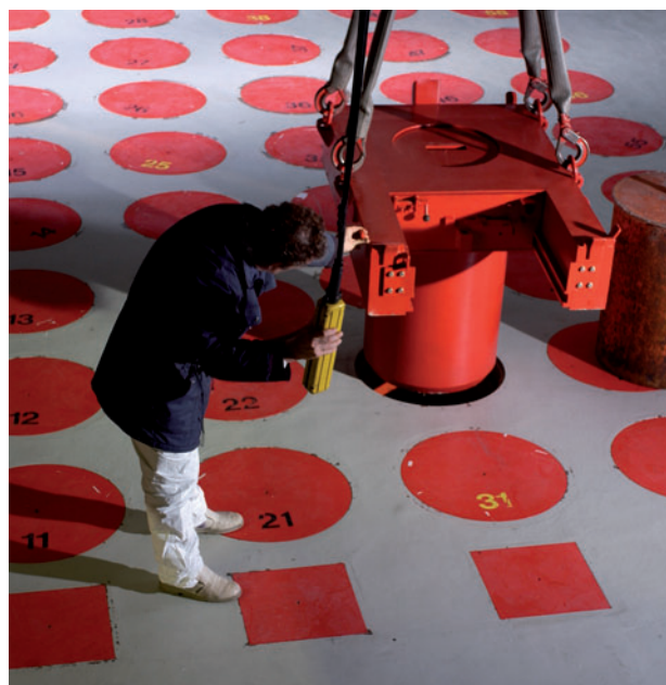
Interim storage hall of BNI 72 (Saclay)
