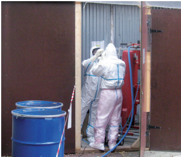
Decontamination of the former Curie laboratories site in Arcueil
