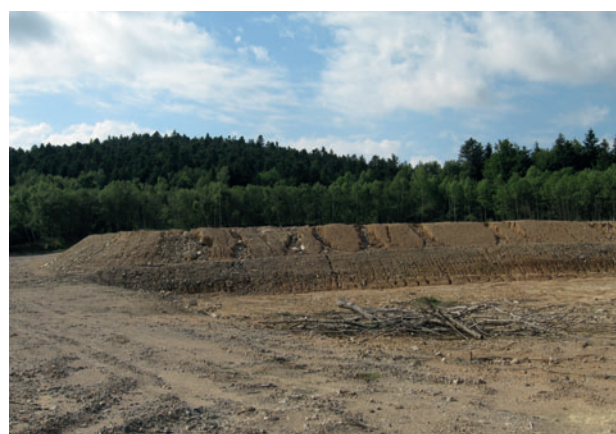
Site of the former Bois Noirs treatment plant (Loire département)
