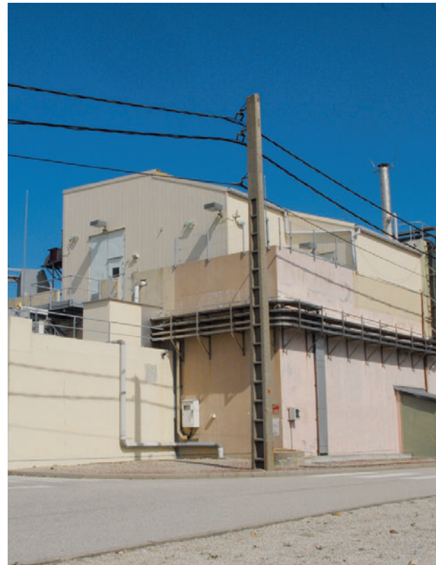
STE2 sludge storage silo
