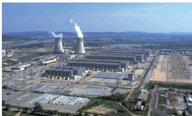
Aerial view of EURODIF, uranium isotopes gaseous diffusion separation plant on the Tricastin site
