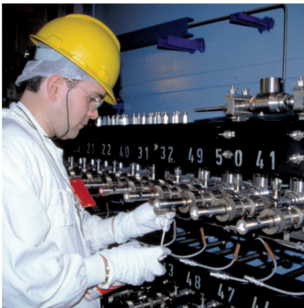
Maintenance intervention by AREVA on the core instrumentation of a nuclear power plant
