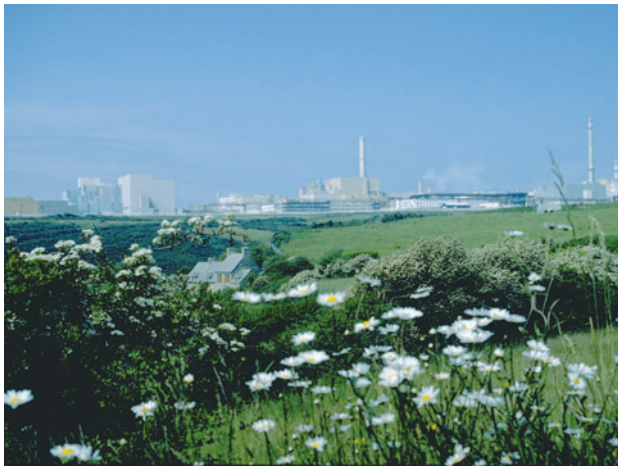
View of the spent fuel reprocessing plant in La Hague
