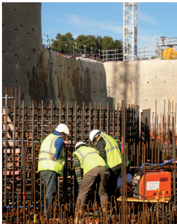
Jules Horowitz Reactor (RJH) worksite in Cadarache – October 2010
