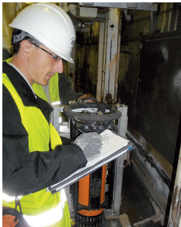
Night-time inspection on the EPR Flamanville 3 worksite – July 2010
