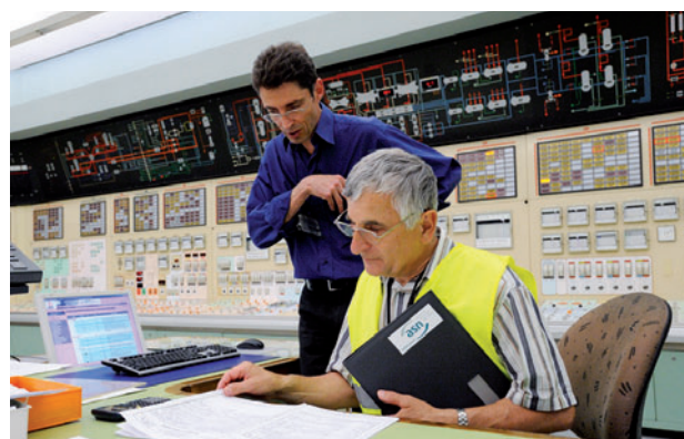
Inspection of the control room during the ten-year inspection of the Tricastin NPP – May 2009
