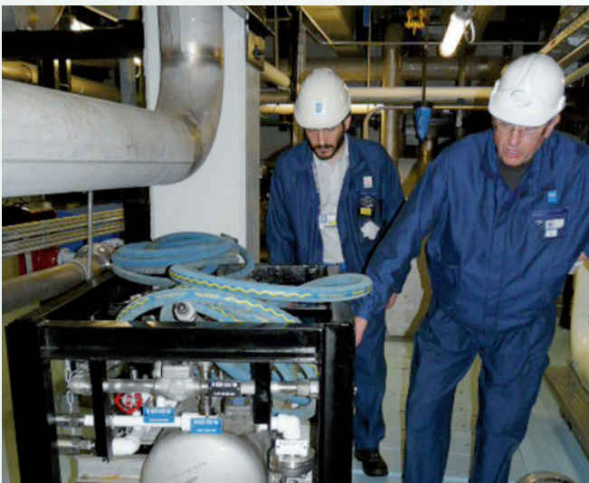
"Environmental" inspection by ASN at the Golfech NPP – April 2010
