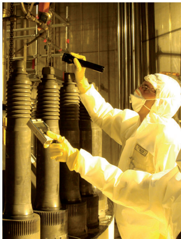
Hydrostatic test during the ten-year inspection of the Fessenheim NPP – December 2010
