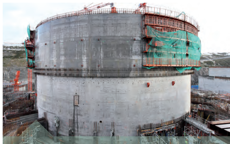
Reactor building, EPR construction site at Flamanville – December 2010
