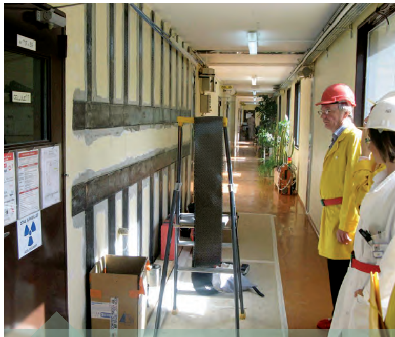
Seismic reinforcement by strips of carbon fibre fabric (TFC) in Cadarache
