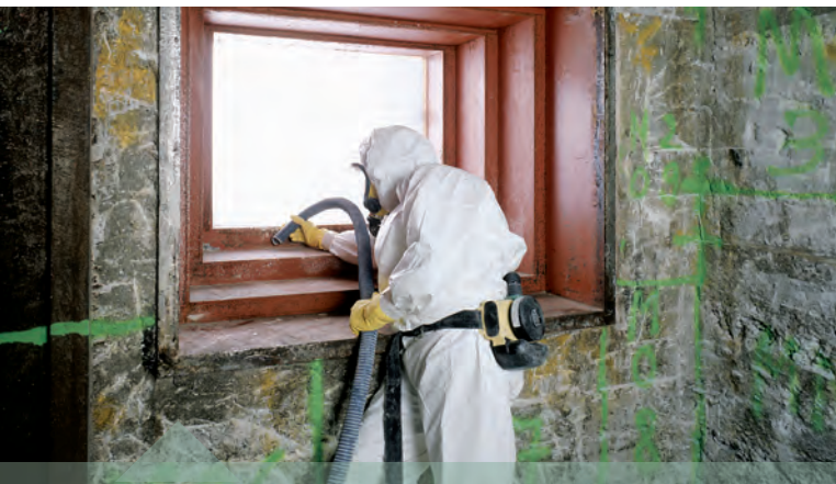
Clean-out of the hot cell of the former TRITON research reactor
