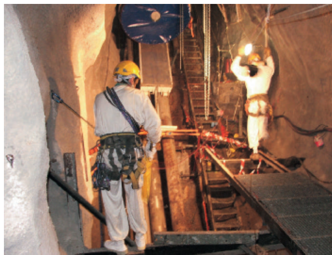
Operators working on decommissioning a ventilation flue on the Chooz reactor
