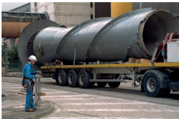
Positioning a cut stack on a semi-trailer during decommissioning of the Superphénix reactor
