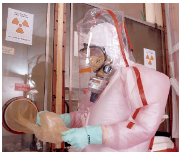
Decontamination of the plutonium chemistry laboratory in Fontenay-aux-Roses by an operator wearing a ventilated vinyl suit with protective breathing apparatus
