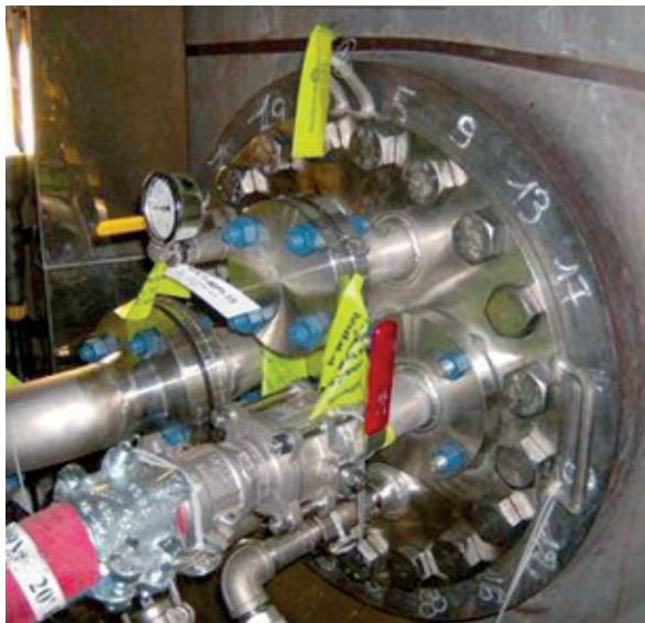
Mechanical plug installed in steam generator tube bundle
