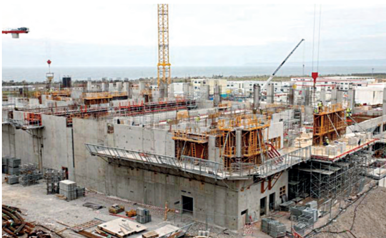
EPR construction site at Flamanville – June 2009: construction of the operation buildings
