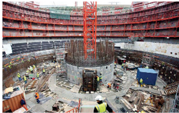
EPR construction site at Flamanville – installation of the nuclear island basemat – September 2009
