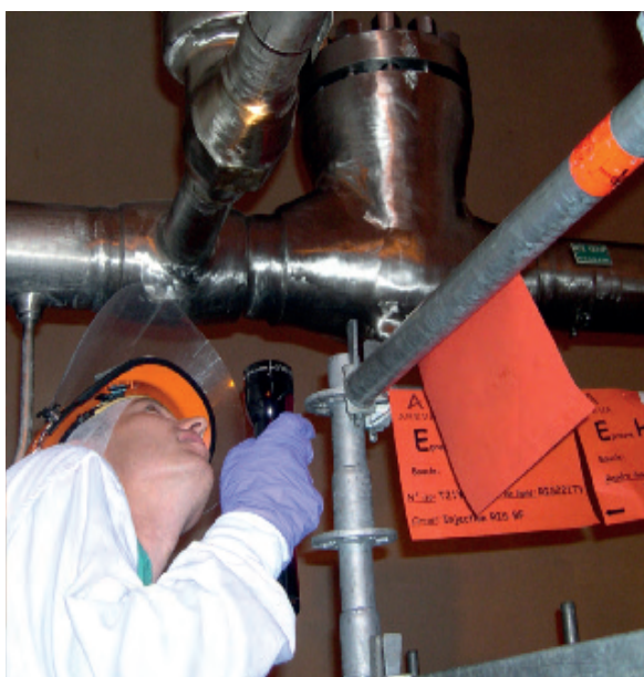
Piping verification by the ASN inspector during hydro-testing of the reactor coolant system (Cattenom in Moselle département) – June 2008
