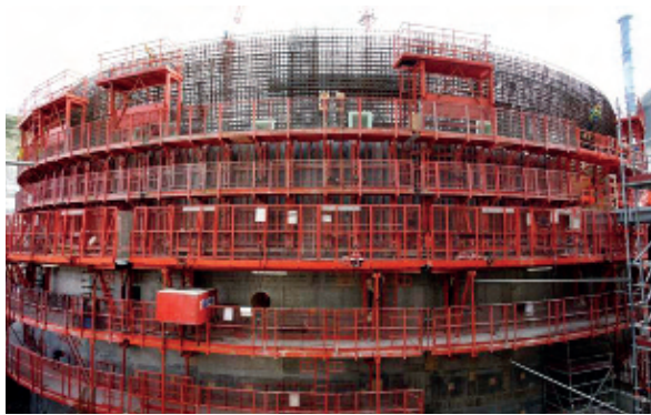
EPR construction site at Flamanville – September 2009: construction of the reactor building outer containment wall
