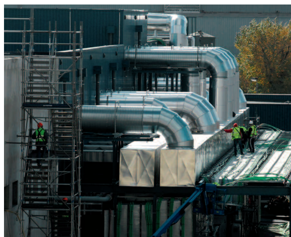
GBII – Construction site at Tricastin
