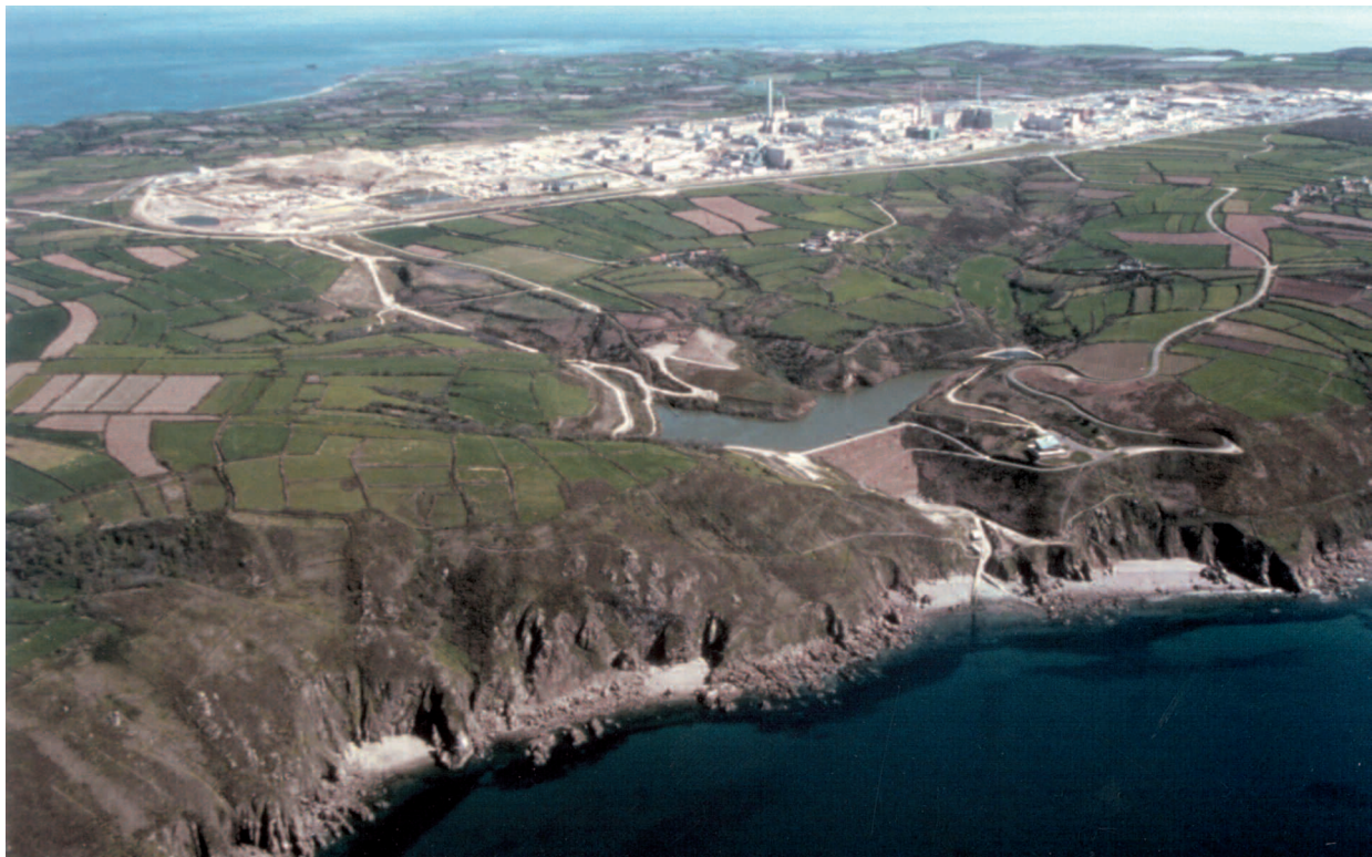
AREVA NC La Hague – Aerial view
