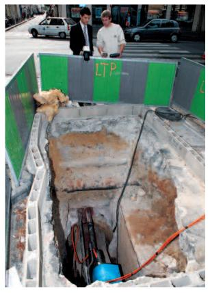
Dose rate check on a gammagraphy worksite during a radiation protection inspection
