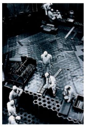
Graphite assembly in graphite gas reactor
