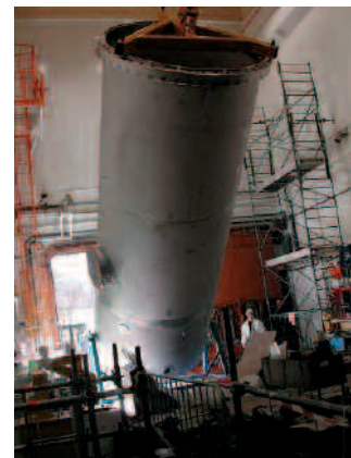
Arrival of the water loop caisson in the CABRI reactor
