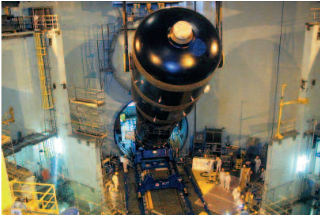
Replacing a steam generator
