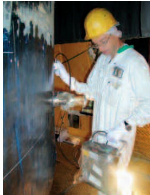
Ultrasound inspection of a welded joint
