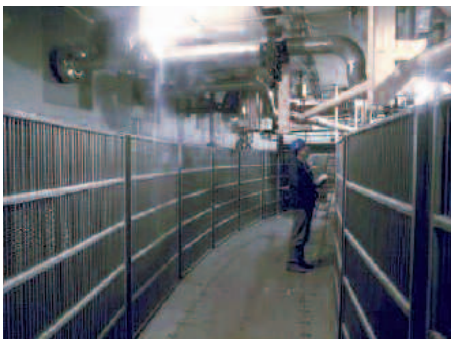
N4 plant series reactor sumps
