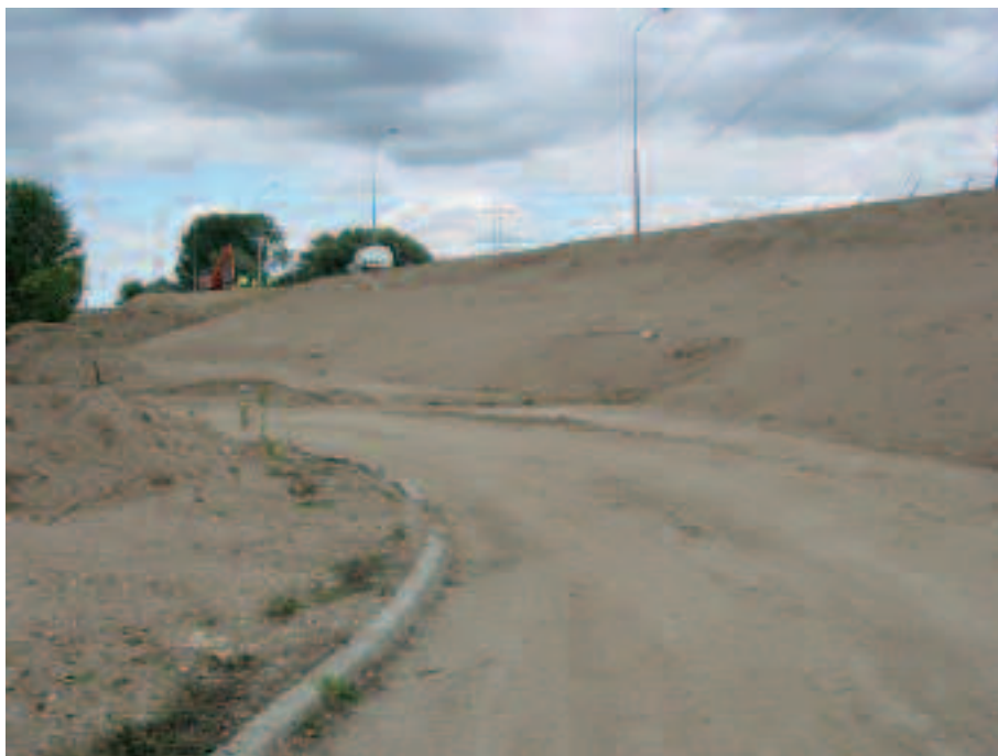
Protective dyke surrounding the Belleville plant (Loire)
