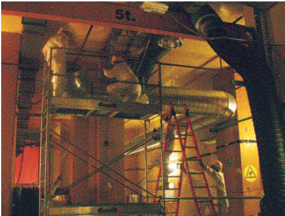
Brennilis – renovation of the ventilation system
