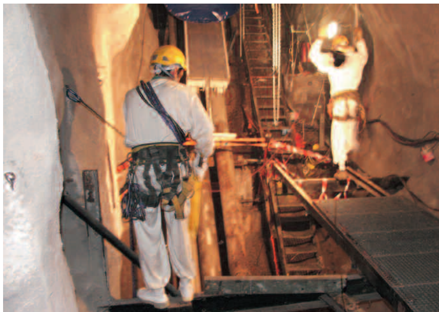
Chooz A – decommissioning of ventilation flue
