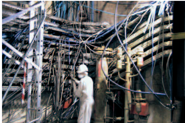
Saint-Laurent – cable removal worksite
