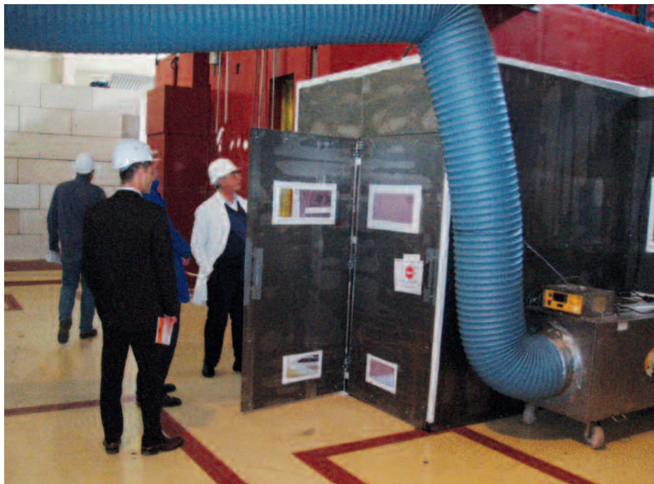
ASN inspection of a bunker installed for decommissioning work on the Strasbourg University reactor on 4 October 2006
