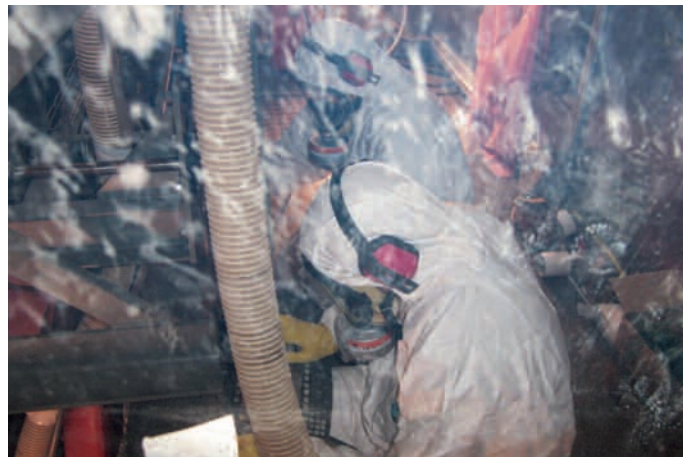
Adjustment of a bush hammering robot (pilot worksite)
