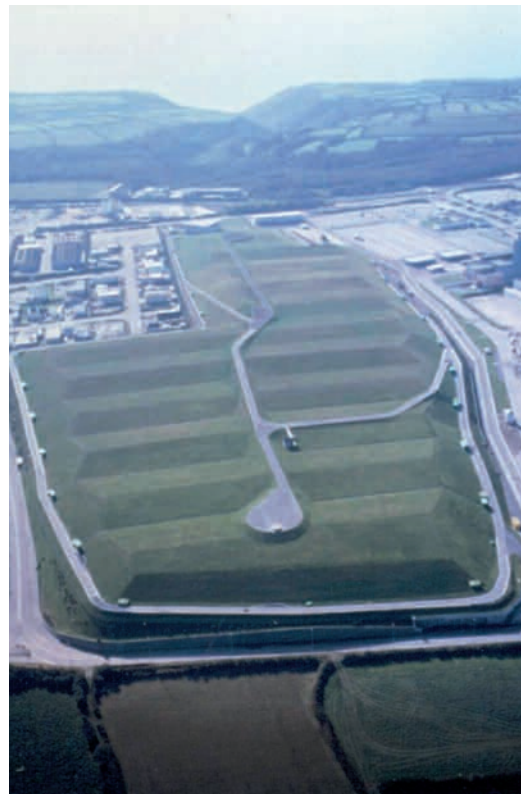
ANDRA – Manche waste repository
