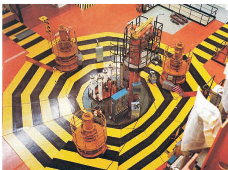
PHÉNIX reactor platform
