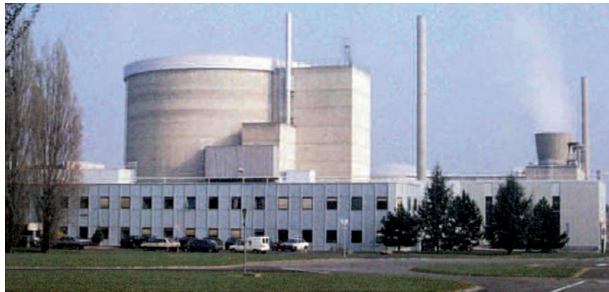
Overview of the ORPHÉE reactor installations
