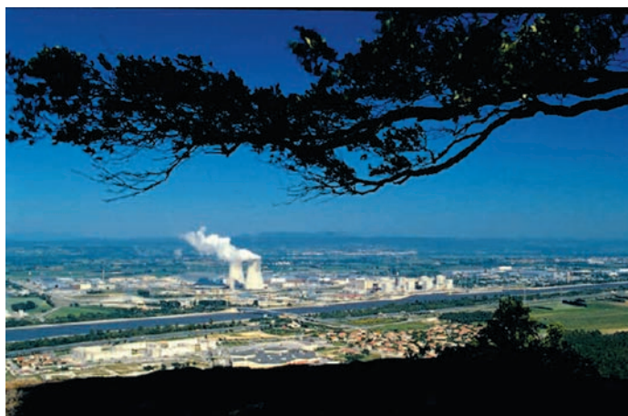
Tricastin site – general view
