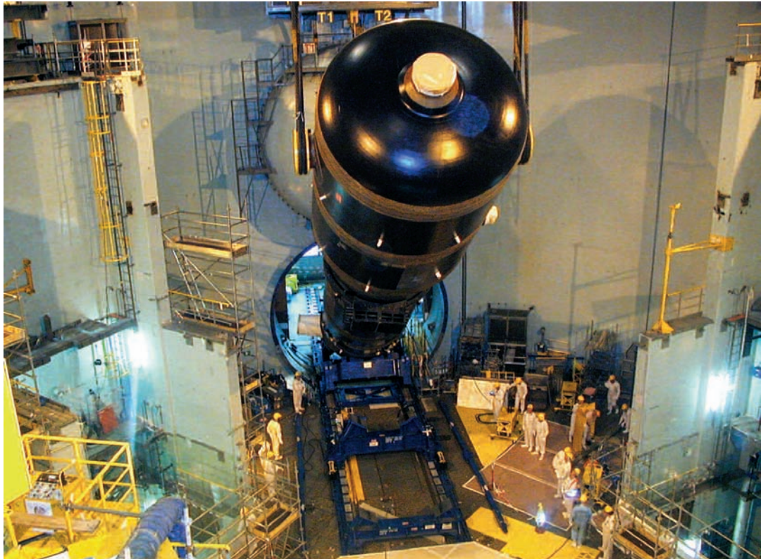
Replacing a steam generator
