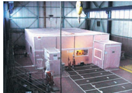
Reactor hall with reactor block cutting hatch – Harmonie
