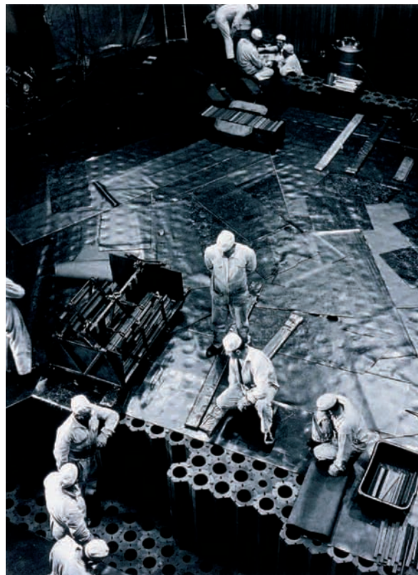
Graphite assembly in graphite gas reactor
