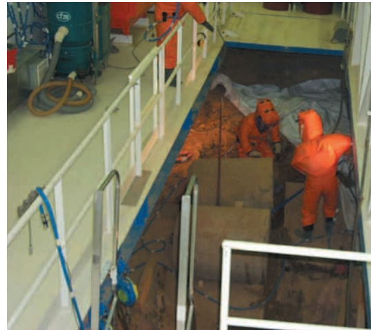
Trench emptying worksite, BNI 56
