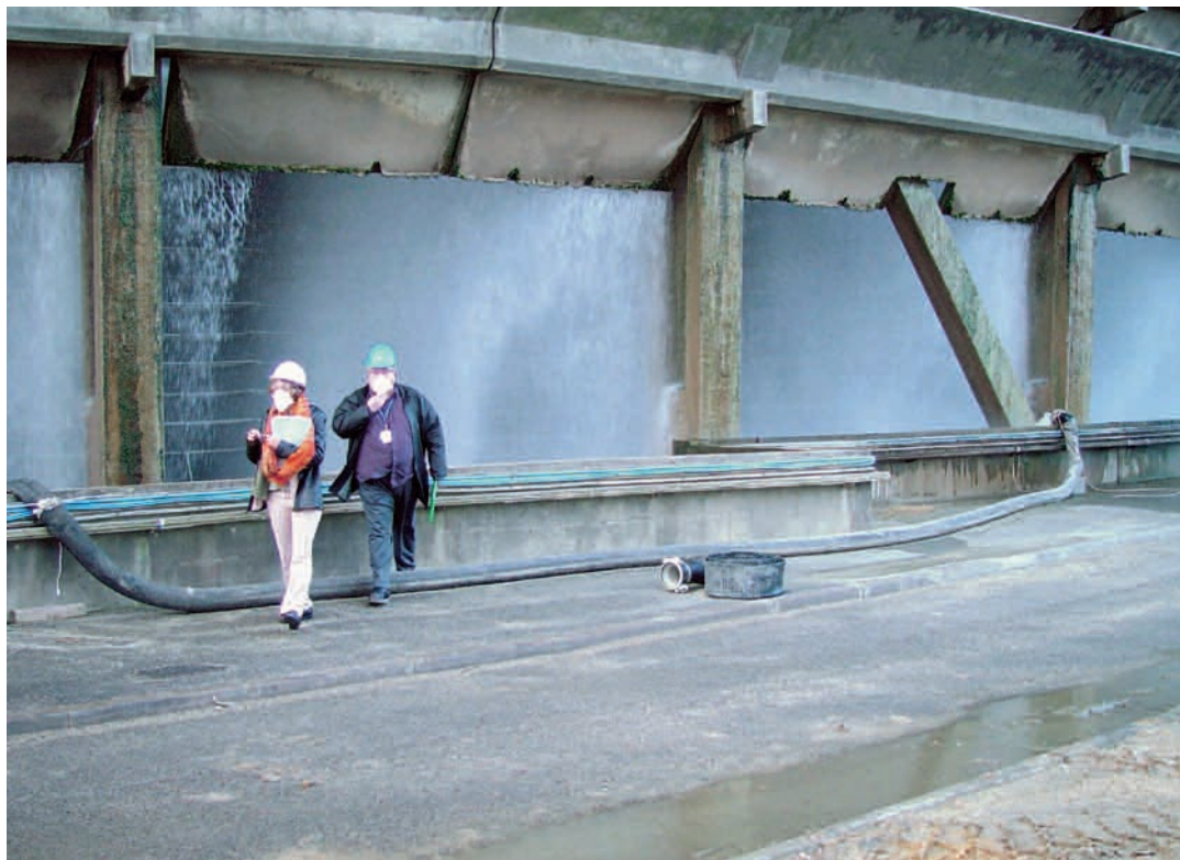
Inspectors checking the cooling towers
