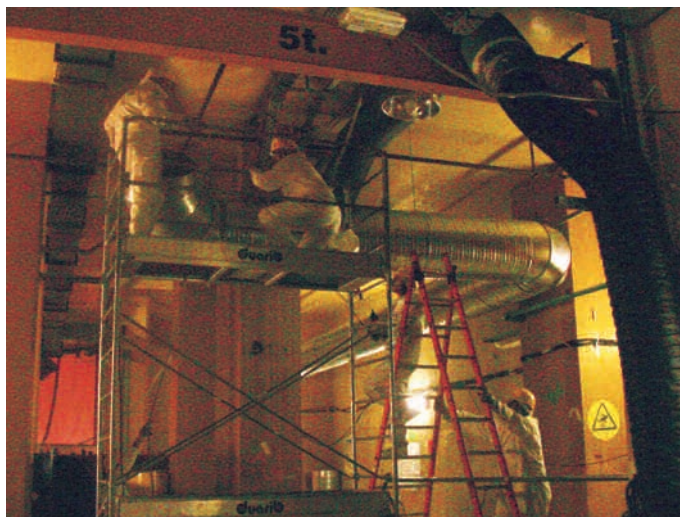
Brennilis – renovation of the ventilation system
