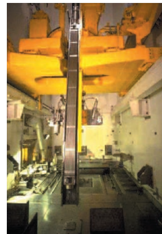
La Hague – T1 shearing and dissolution shop supply cell
