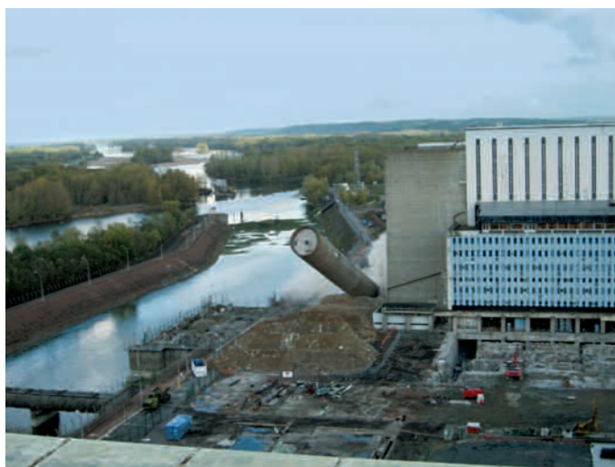
Chinon – blasting of the CHA 3 water tower
