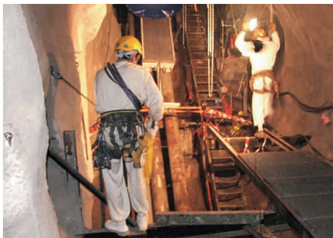
Chooz A – dismantling of ventilation flue
