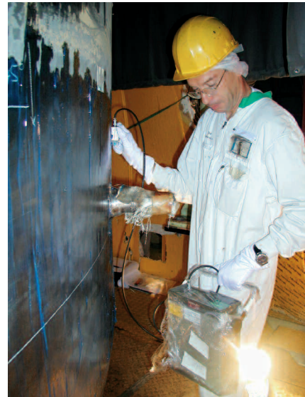
Ultrasound inspection of a welded joint
