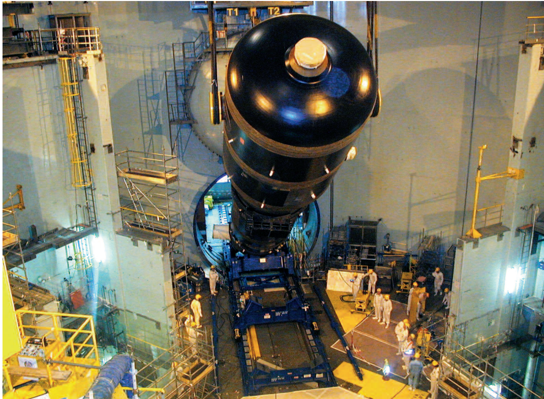
Replacing a steam generator
