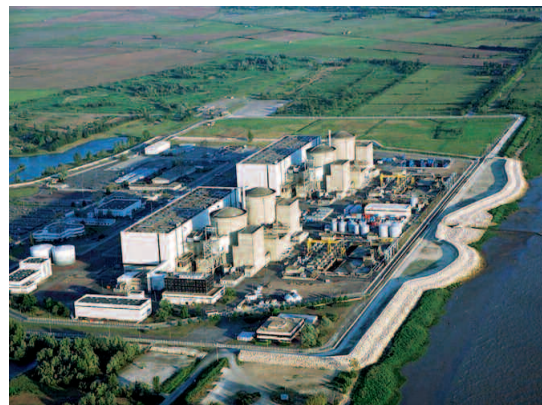
Protective dyke surrounding the Le Blayais plant (Gironde)
