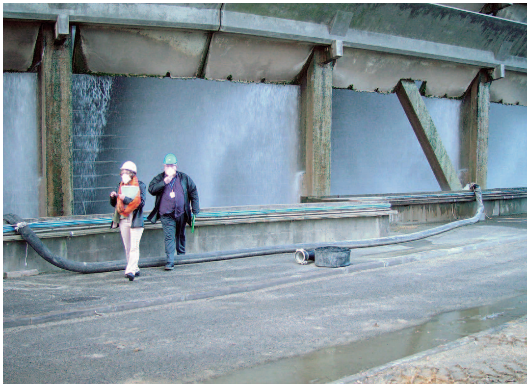
Inspectors checking the cooling towers
