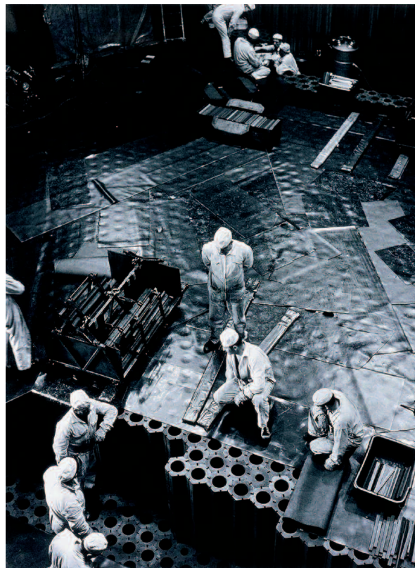
Graphite assembly in graphite gas reactor
