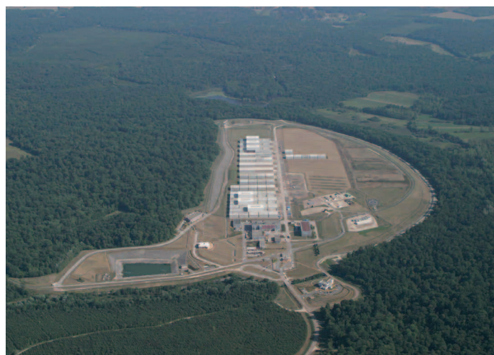
ANDRA – Aube waste repository
