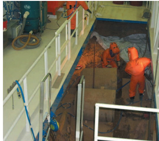
Trench emptying worksite, BNI 56
